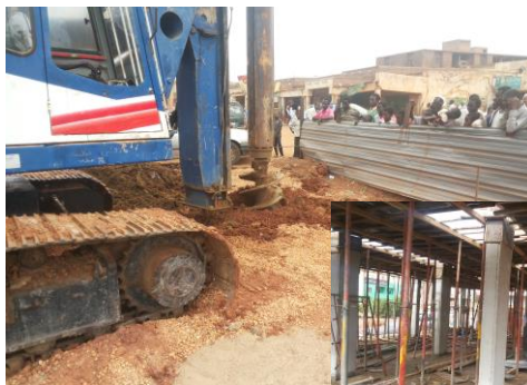
Commercial Farms Bank - Sennar Branch(Site manager, construction work as Acts of deep Foundations & CUP
